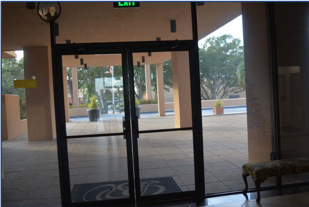
Photograph No. 2: Common element doors include the front entry, fire doors, and other access doors to the building. These have to be in the reserves.
