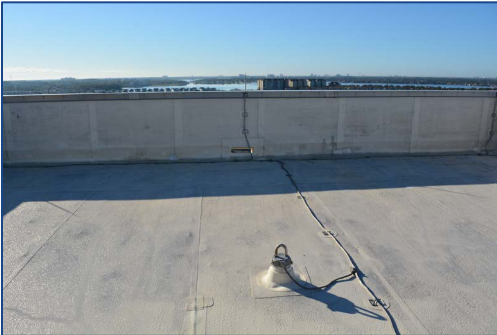
Photograph No. 6: The TPO roof covering is in good condition and its cost shared among the unit owners.
