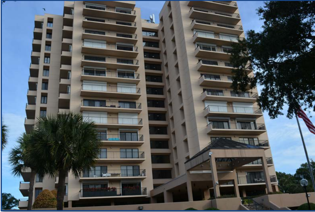
Photograph No. 1: The Bayview Reserve building is 15-stories and currently has good coatings.
