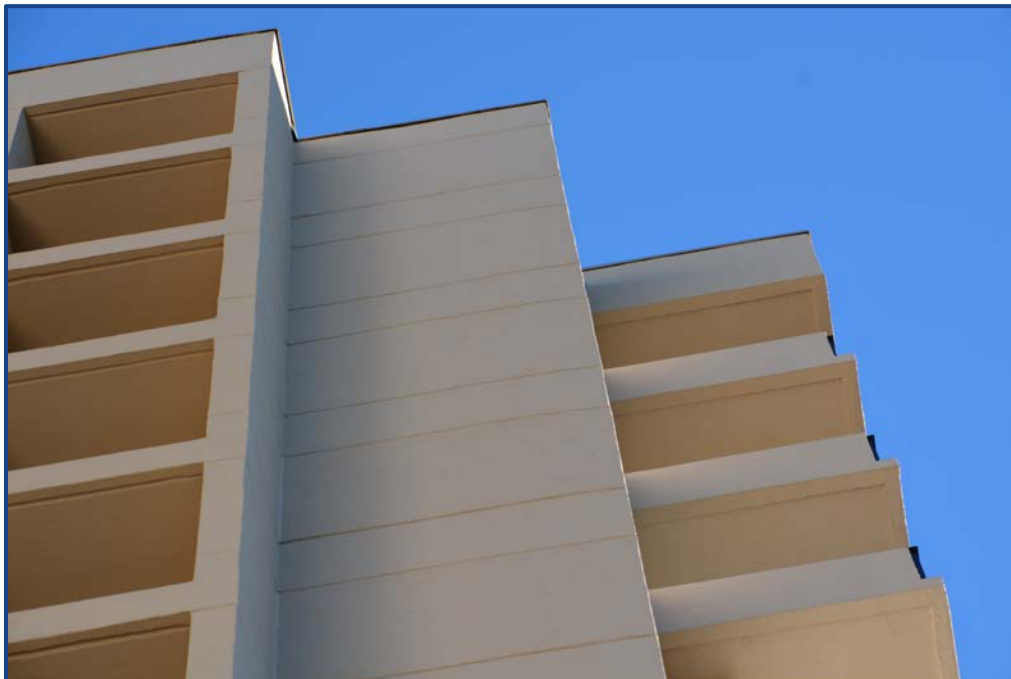
Photograph No. 8: Building waterproofing and painting are to be performed every 7 to 10 years.
