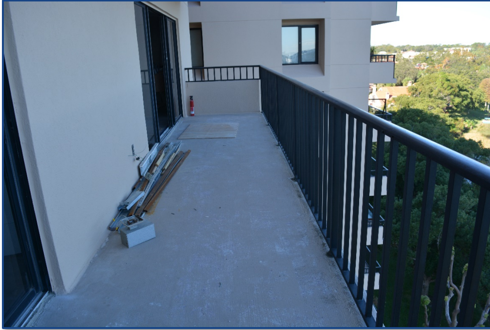
Photograph No. 9: Waterproofing the decks each decade is important to maintain structural integrity of the balconies and guard rails.
